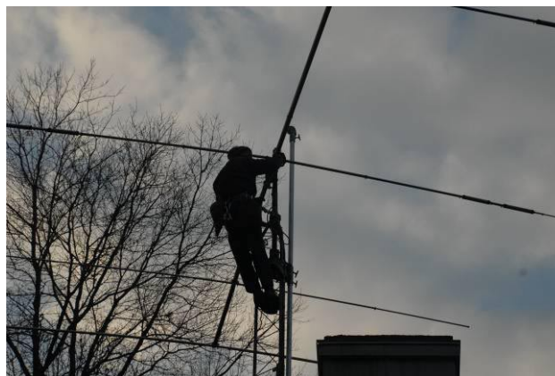
Ralph KD1SM removing the antenna from the tower.
