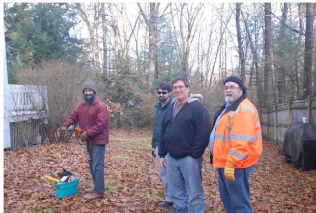
Tower crew ready for second tower take down; KD1SM, N1QDZ, K1BG, KK1X, KB1ESR (behind the camera).
