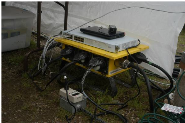
PDU and network switch - Photo courtesy Jim N8VIM
