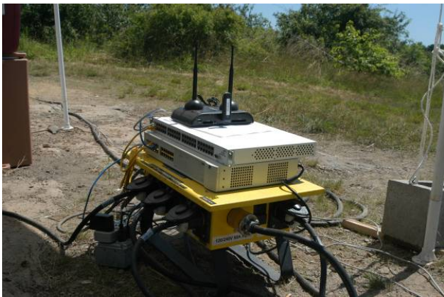
Power, Networking and Internet – Photo courtesy Jim N8VIM
