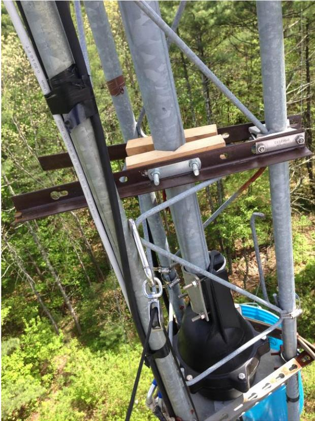
Above is the fixture built and used for the rotator replacement. While the device worked as planned a couple of issues were identified. The fixture had many loose parts with two U-bolts, nuts, and closing plates as well as two sets of saddle clamps. So one improvement was to capture the closing plates and saddle clamps to the angle iron. The second issue was the angle iron ends being a bump hazard so they were protected with rubber cushions.
