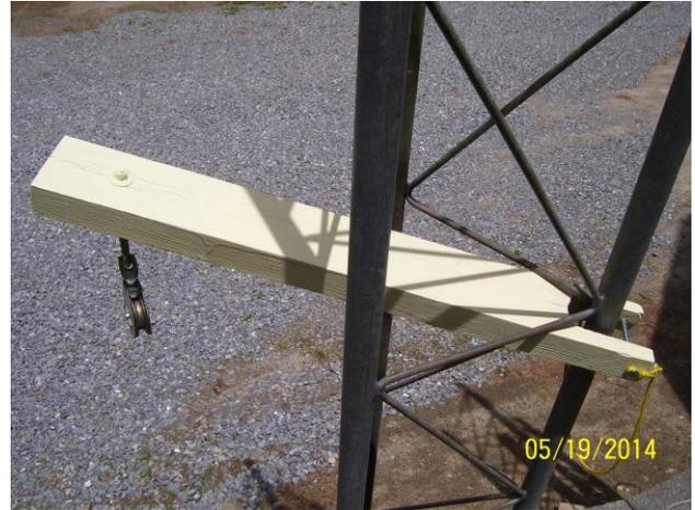
The solution was an outrigger that is secured to one tower leg and is grooved to match the rung that it sits on both of which keep it from moving. It is not intended to support heavy loads but things like a tool bucket or rotator.
