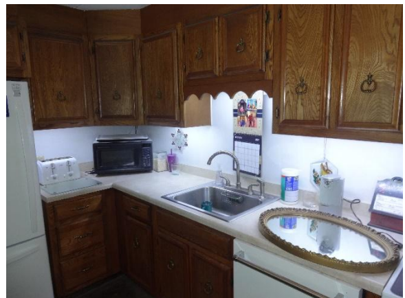
(The mirror lying over the dishwasher was the technique I used to see how I was placing the LED strips. Once you stick them on there is no moving them and, since they are a flat strip, they don't flex. So you want to make sure you place them properly—once!) KD1LE photo
