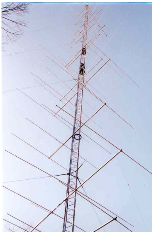
Stacks of 10 & 15m 4-element yagis
