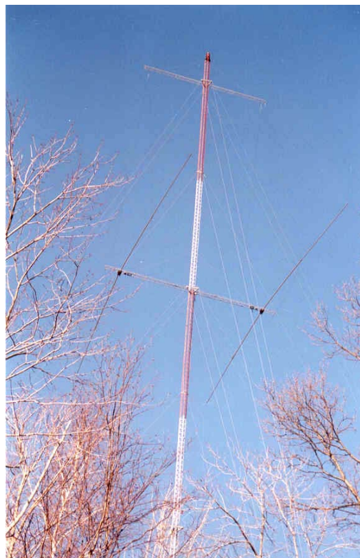
The 80m tower and upper phased delta loops
