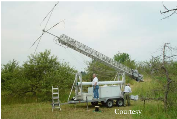
Once installed on the mast (and cables connected) the tower is rotated vertical before extending it. All the guys for the tower and halyards for the dipoles and ZL Special are installed and draped to the rear of the trailer and can be seen under the tower.
