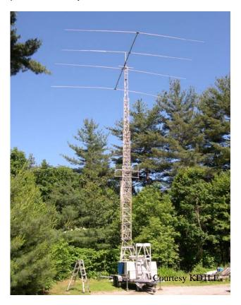
Since the antenna boom of the 20 meter antenna is too long to be put on the mast when the tower is horizontal it had to be mounted in two pieces. The purpose of these tests was to confirm the assembly procedure and antenna performance. The motto heard there was "If it hasn't been tested it doesn't work." It worked fine at Field Day so the test was successful.
