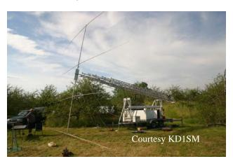
A particular challenge for the 20 meter yagi antenna is that its boom is too long to mount it on the tower mast with the tower horizontal. So the back ¾ of the antenna are mounted and then the tower tipped up slightly so the front part of the boom and the first director can be attached.
